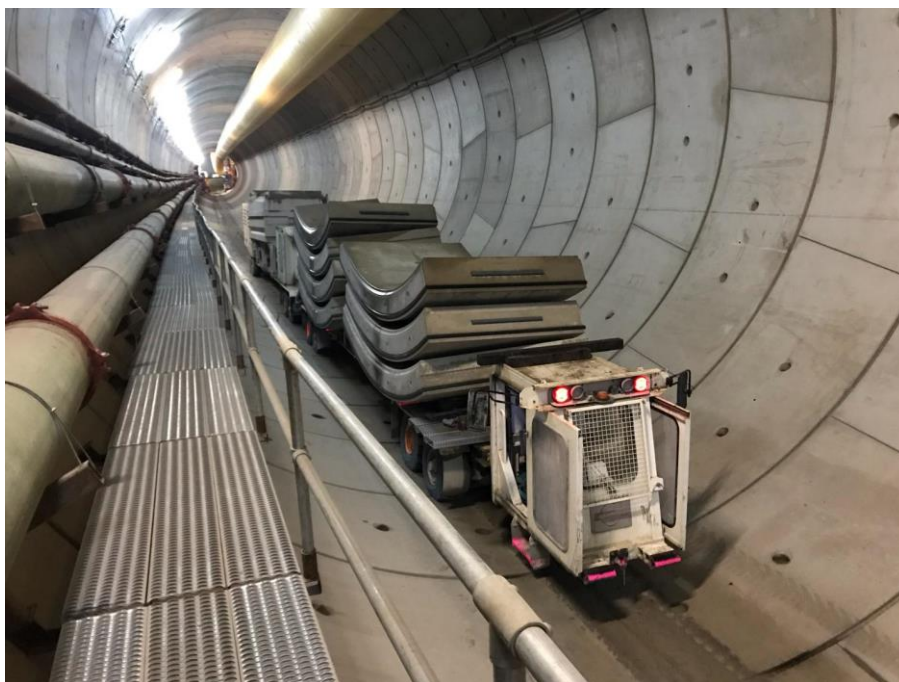
The 70-ton TSP transporting segments
